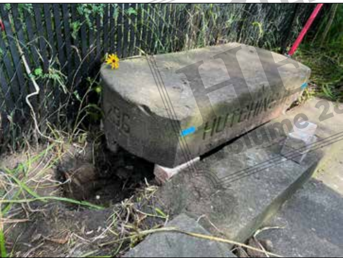
The block is jacked up prior to inserting fill underneath.
